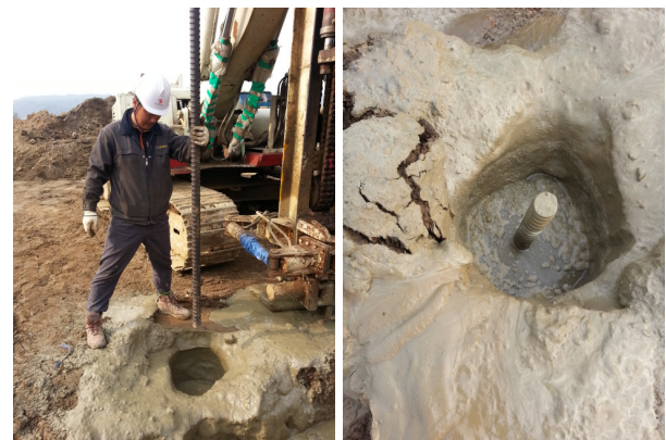
(c) Inserting a reinforcement
