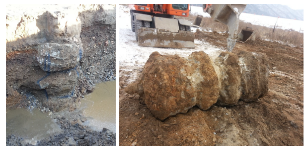
(a) Site excavation
