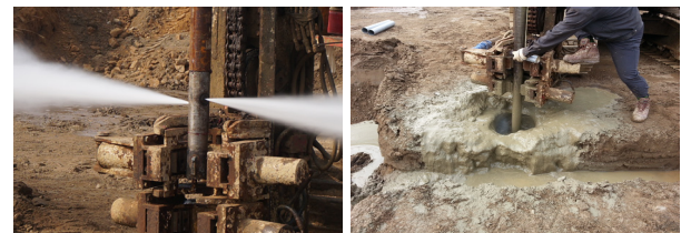
(a) Ground boring
