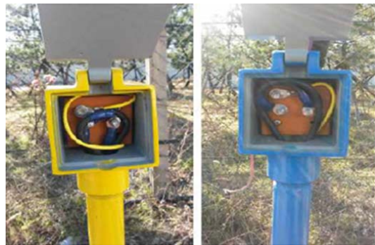
Fig. 11. Test Boxes which have leds(yellow color line) of solid reference electrode.
