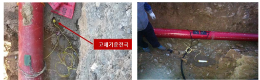
Fig. 7. Installation of reference electrode near pipe.
