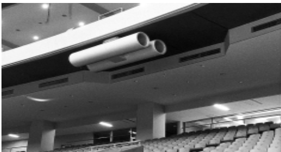
〈Fig. 2〉 Air-circulation fan and diffuser in Nagoya Dome
