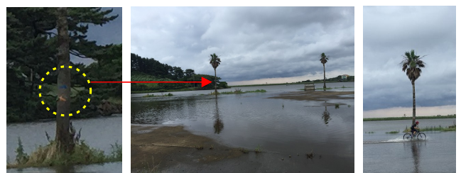
Figure 6. Problem with the site of a route sign
