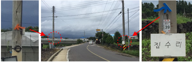
Figure 7. Inconsistency in the installation of a route sign
