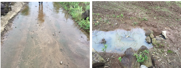
Figure 14. The road uncomfortable for walking due to soaked in water
