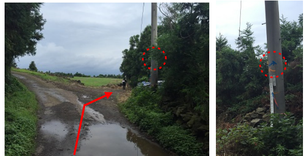
Figure 5. A route sign on an inappropriate spot at a crossroads
