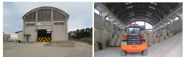
Figure 7. Snow control material storage of the highway
