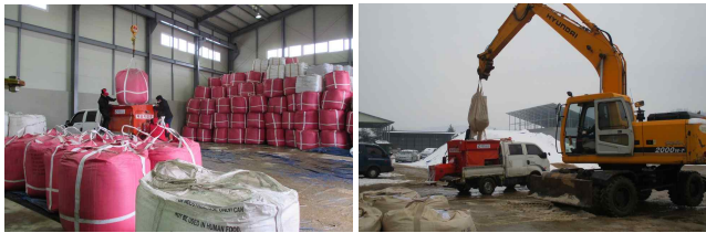
Figure 2. Operations loading salts
