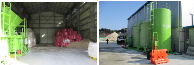
Figure 6. Snow control material storage : Case B
