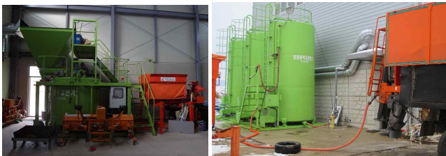
Figure 3. Operations mixing and injecting the salt brine
