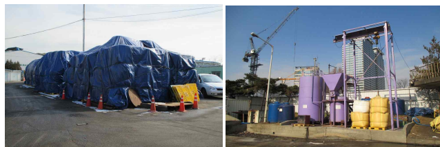
Figure 4. Outdoor storages(left), brine mixer, and tank(right)
