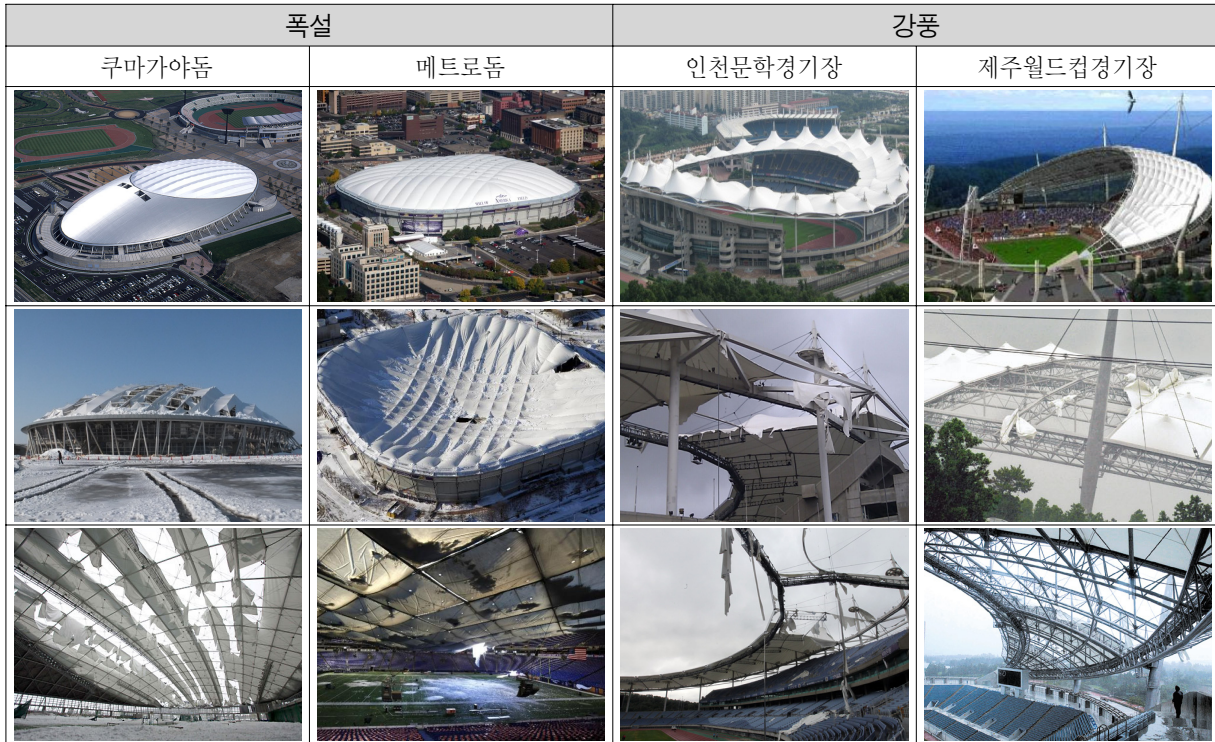
〈Table 2〉 Real cases of collapse of membrane structures
