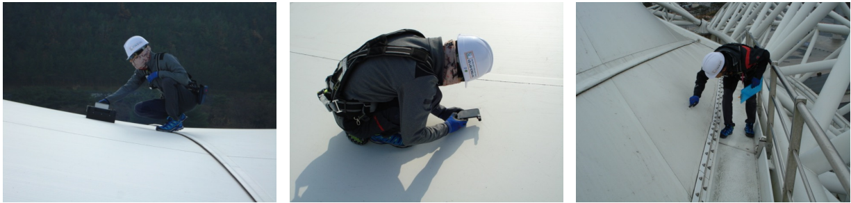
〈Fig. 1〉 Author under maintenance on the Daegu Stadium
