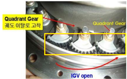
Fig. 9. Stuck of Quadrant Gear
