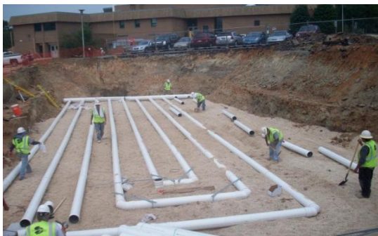
Fig. 1 A case of earth tube system ( http://www.homeintheearth.com/ )
