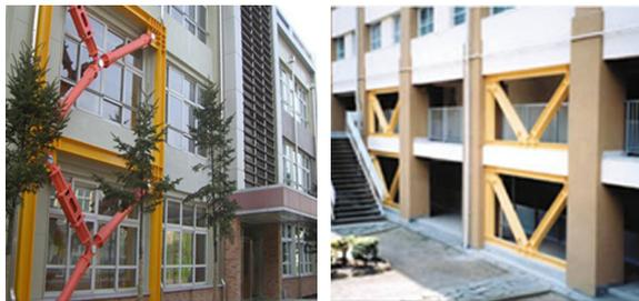
Fig. 1. Examples of typical bracing damper system.
