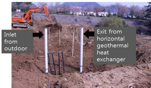
Fig. 4 Inlet and Exit location of system.
