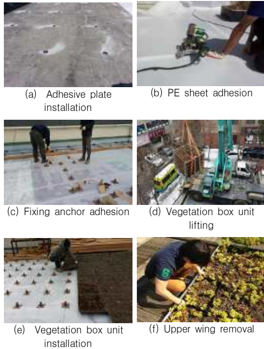
Figure 4. Construction process of vegetation box unit system
