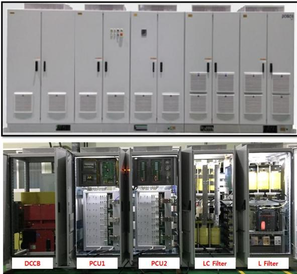
Fig. 14. System constitution of battery simulator #2.
