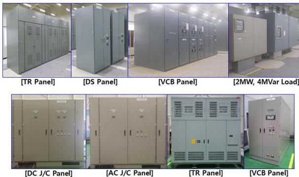
Fig. 23. Facilities for grid connection, EUT connection, load test.
