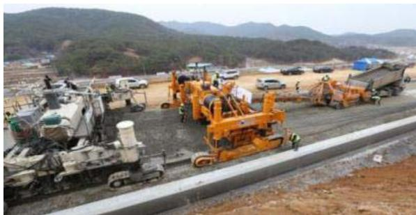
(b) Reinforcement Placing and Concrete Paving
