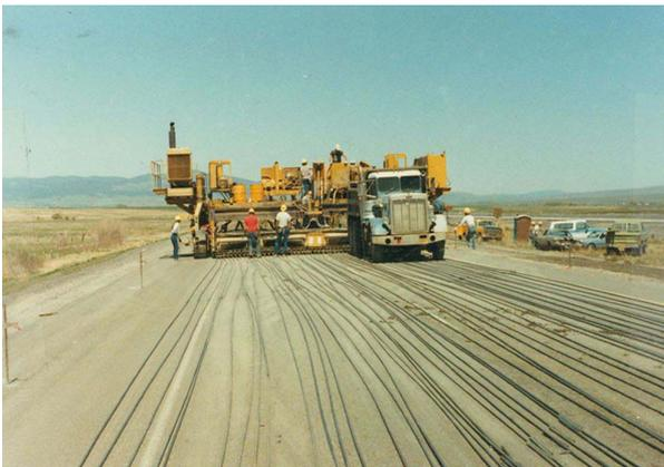
Fig. 4 Concrete Paving by Feeding Concrete Material in Front
