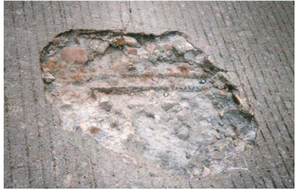
Fig. 5 Pavement Distress by High Steel
