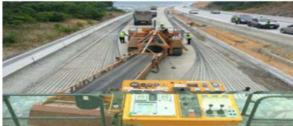
(a) Connecting Reinforcing Steel and Starting Concrete Paving
