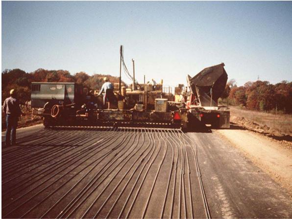
Fig. 3 Front View of the Field Application of Tube-Feeding Method
