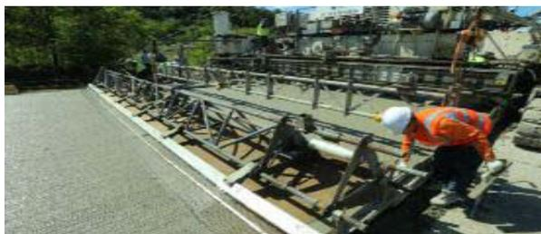
(c) Arranging Surface and Tining After Concrete Paving
