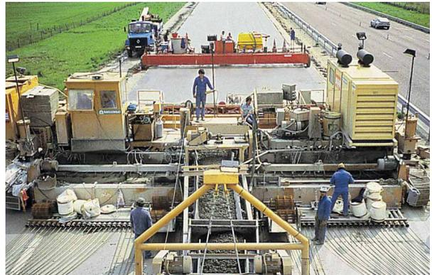
Fig. 6 CRCP Construction with Mechanical Tube-feeding Method (France)
