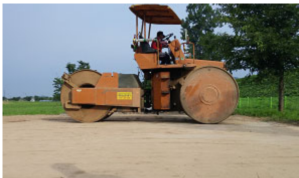
Fig. 9 Backfilling and Compaction
