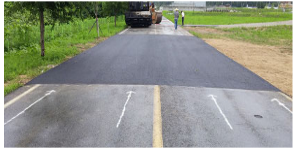
Fig. 10 Asphalt Paving and Compaction
