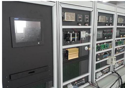
Figure10. Wind-PV hybrid control system
