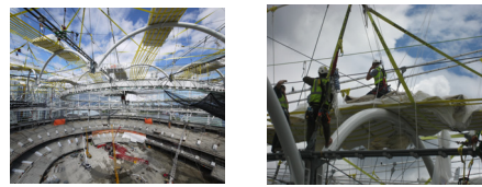
<Fig. 8> Install of roof membrane
