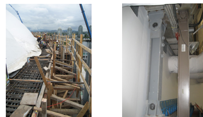
<Fig. 4> Concrete transfer beams and support columns
