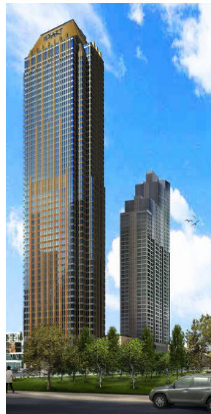
Figure 5. Grand Hyatt Metrocenter, Manila. Image copyright Federal Land Inc.
