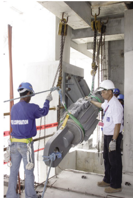
Figure 4. installation of dampers for St Francis Shangri-La Place. Image copyright Arup.
