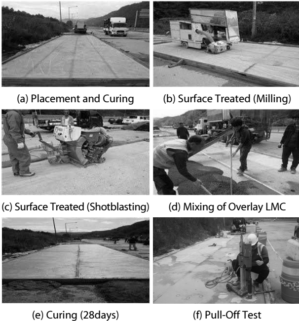
Fig. 1. Process of Bonded Overlay on Concrete Slab
