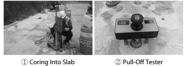
Fig. 5. Process of Pull-off Test
