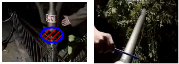
Figure 9. Lack of safety measures(안전조치 미흡)
