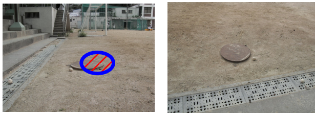
Figure 7. Exposed manhole(노출된 맨홀)
