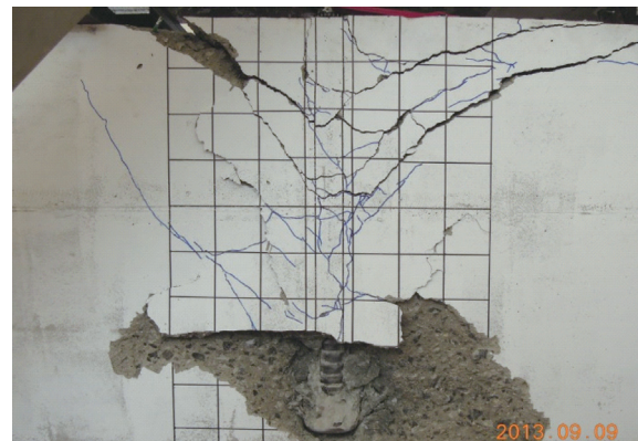
(a) Side-face blowout failure of Beam-column joint test
