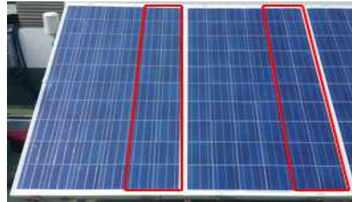
Fig. 8 PV module installed in outdoor
