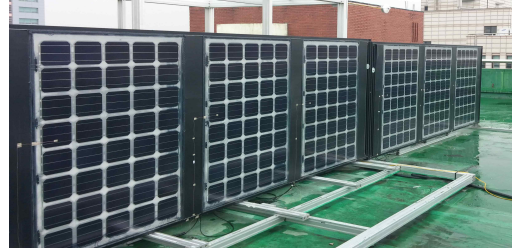
Fig. 6 Picture of the BIPV system installation
