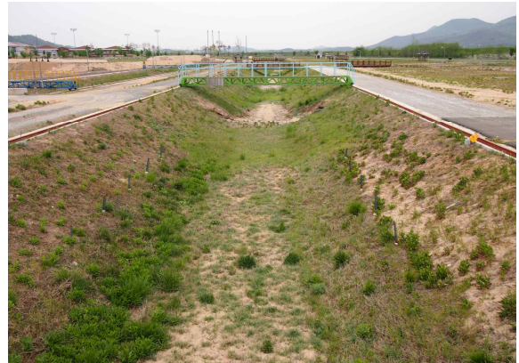
Fig. 3. Bedform of Straight Channel
