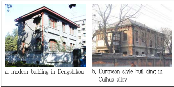
Figure 9. Demolition of buildings[16]
