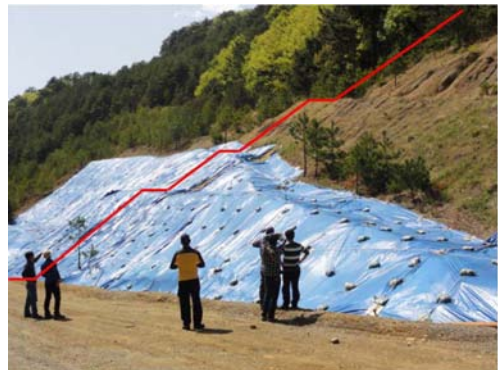
Fig. 1. Location of waste-dump slope for numerical analysis.
