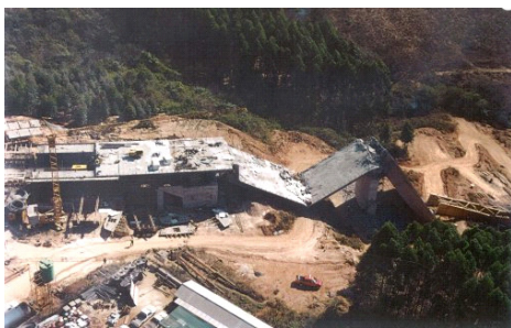
(b) Injaka Bridge
