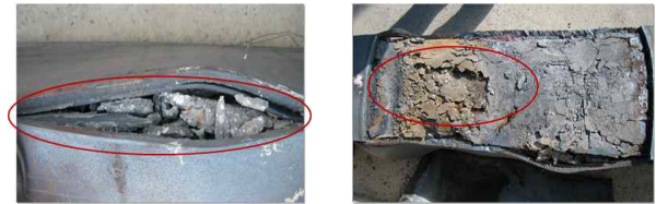
Figure 2. Failure of CFT after 2 hours fire test in previous test
