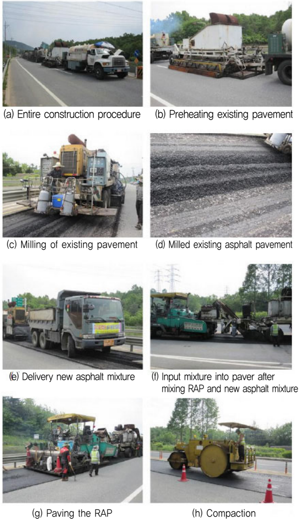
Fig. 1 HIR Field Construction (Kwon et al., 2013)
