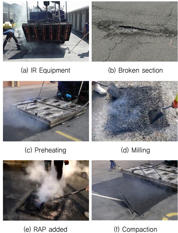
Fig. 2 Repair Work Using of Infrared Equipment (KAIN INTL, infrared patching)
