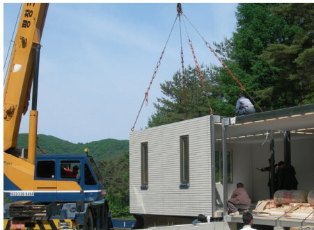
(b) Installation of Unit Module
