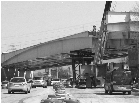
Fig. 3 Arch-type Composite Girder
