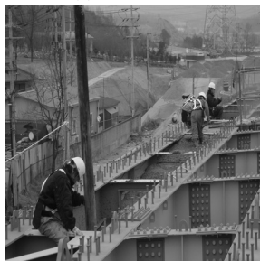
(c) arch concrete casting
