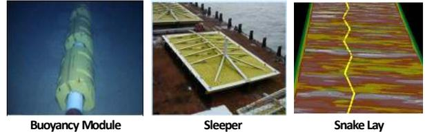
Fig. 4 Global Buckling Control Methods
