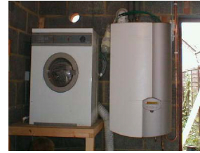
Fig. 7 Cogeneration system with Stirling engine/alternator(Microgen)
