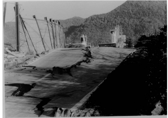
Photo. 1. Rising of Road
