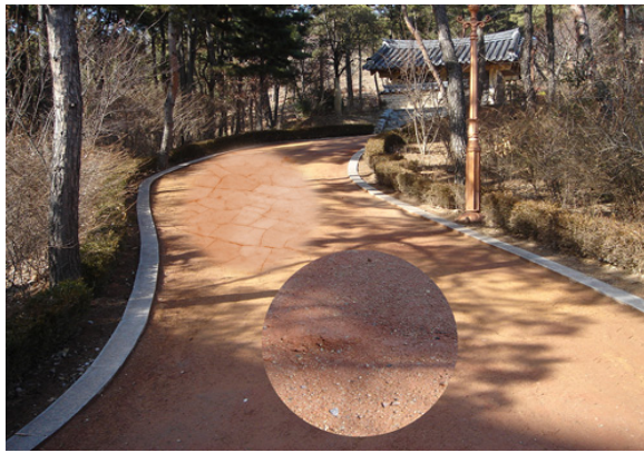
Fig. 1. Crack and pothole of loess road
