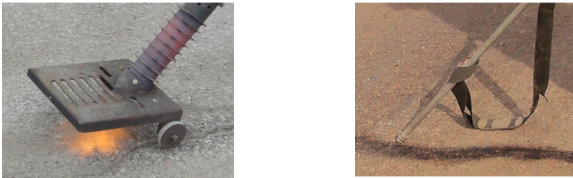
FIGURE IV ADDITIONAL CRACK CLEANING DEVICES: HEAT LANCER (LEFT) AND AIR BLOWER (RIGHT)
