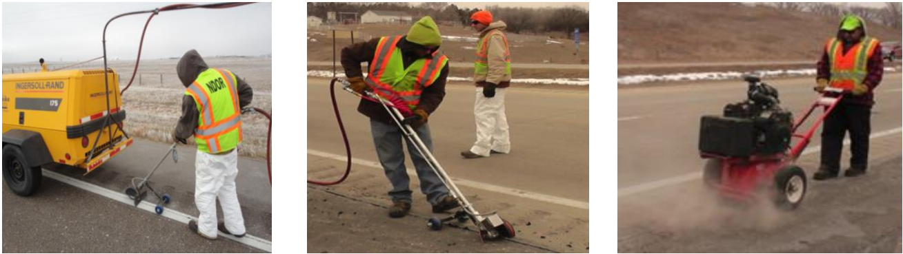
FIGURE III FIELD TESTS WITH THE NDOR ON CCD (LEFT AND MIDDLE) AND ROUTER (RIGHT)
