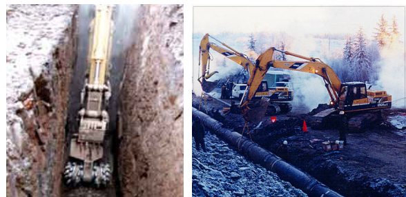
a) Extreme technologies for construction machinery
