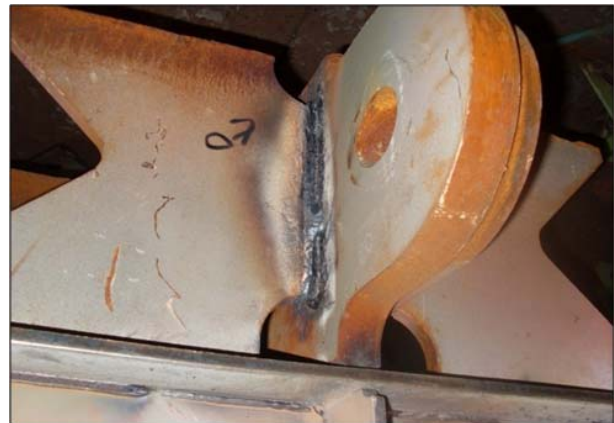
(b) Lug hole and double plate
