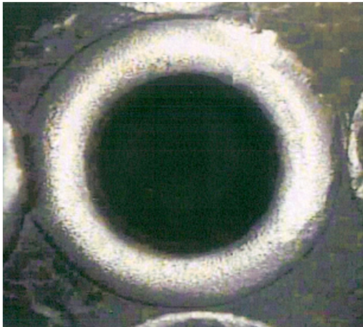
Fig. 7 Visual inspection for Tube End Sleeved Welding
