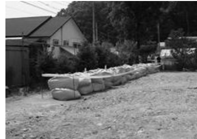
(k) Construction completion
