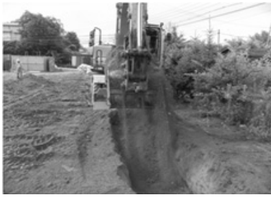
(a) Bed excavation
