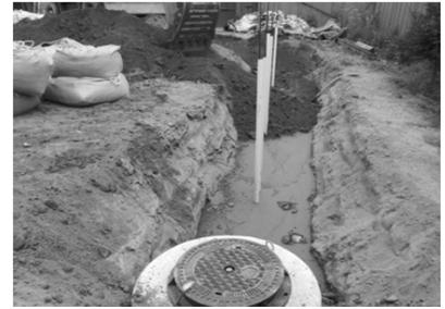
(i) Laying a backfill material at the top
