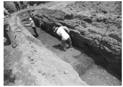
(c) Laying a sand at the bottom
