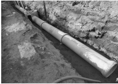
(g) Laying a sewer (backfill material)
