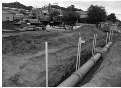
(h) Installing settlement gage
