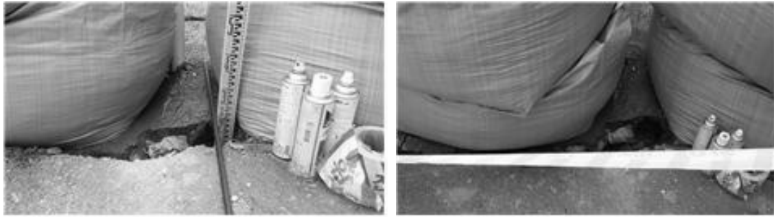
Fig. 11. Ground settlement in sand compaction area
