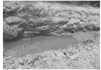
(f) Laying a backfill material at the bottom
