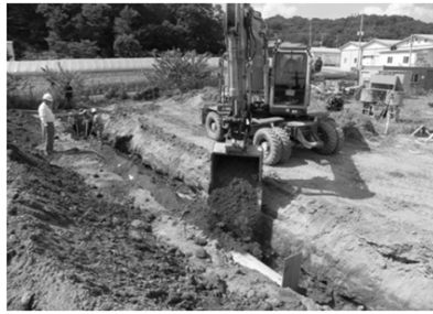
(e) Laying a sand at the top (sand compaction)
