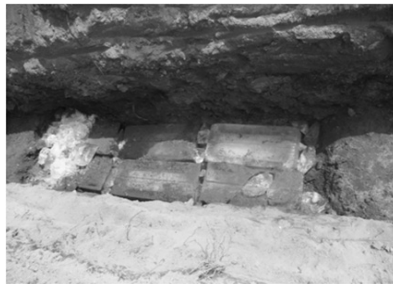
(b) Laying a ice block at the bottom
