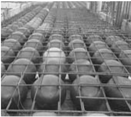
Fig. 1 Voided slab with ball-type voiding material
