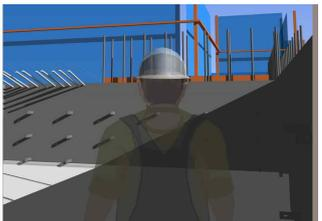
Figure 10. Protruding rebar and metal pin
