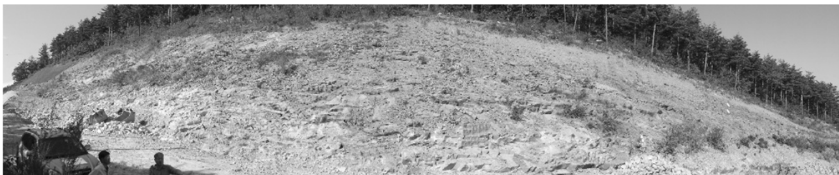
Fig. 4. The condition of the slope of interest
