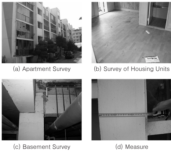
Fig. 3. Site Survey for Deconstruction
