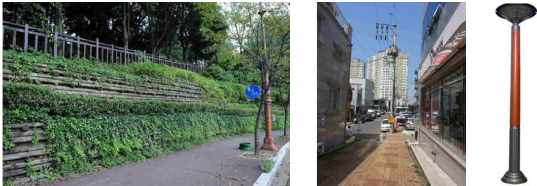
Fig. 5. Existing iron street lamp, ground current split factor, and wood street lamp.
