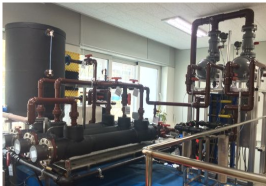
Fig. 2 Experimental equipment of VMD system
