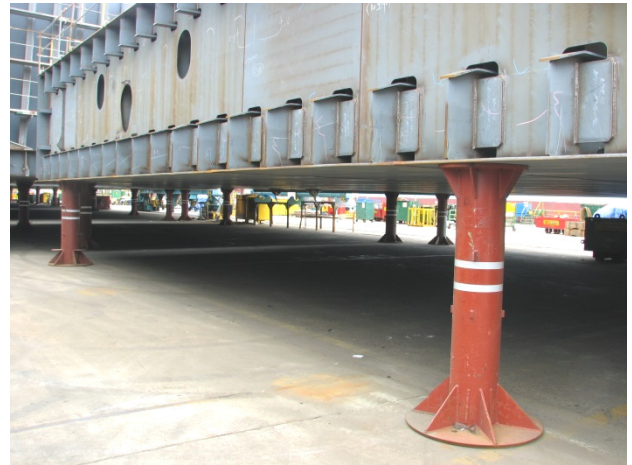
Fig. 5 Erection face of block
