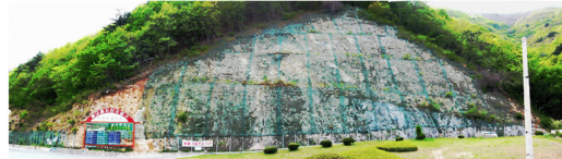
Fig. 4. Photograph of slope-1.
