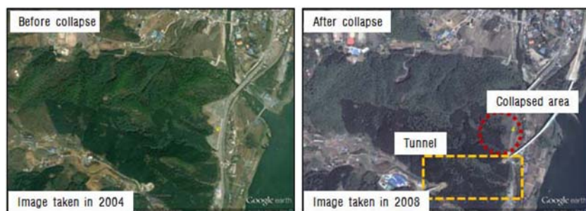
Fig. 2. Slope failure in area B.
