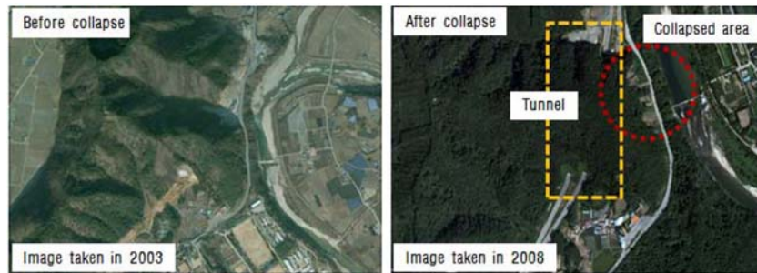
Fig. 1. Slope failure in area A.
