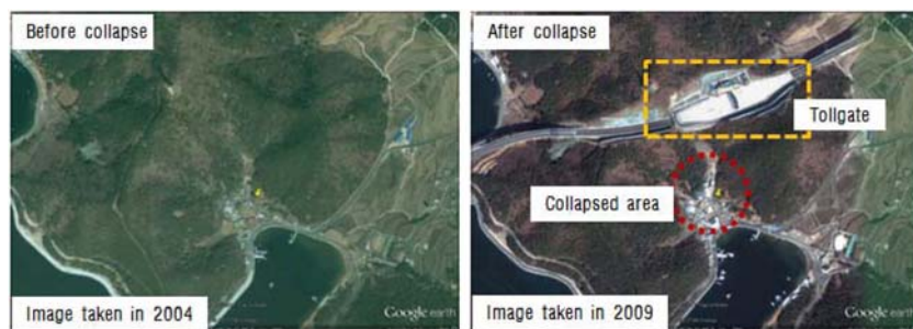
Fig. 3. Slope failure in area C.
