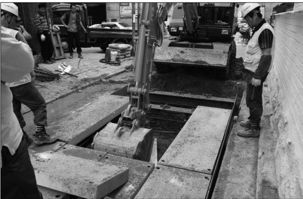
Fig. 21 Pipe Construction through Opening Composite Lining Board
