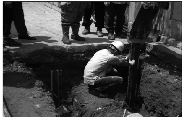
Fig. 18 Installation of Steel H Piles by Excavator
