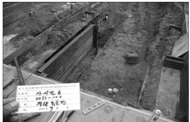
Fig. 19 Installation of Composite Retaining Walls
