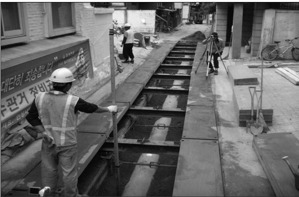
Fig. 22 Pipe Level Test after Pipe Installation
