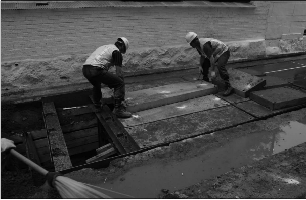
Fig. 20 Placement of Composite Lining-Board
