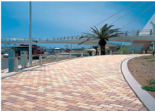
Fig. 4 Photocatalytic Block Pavement in Japan
