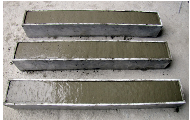
(c) Concrete Placing
