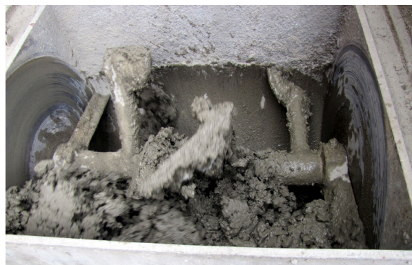
(b) Concrete Mixing
